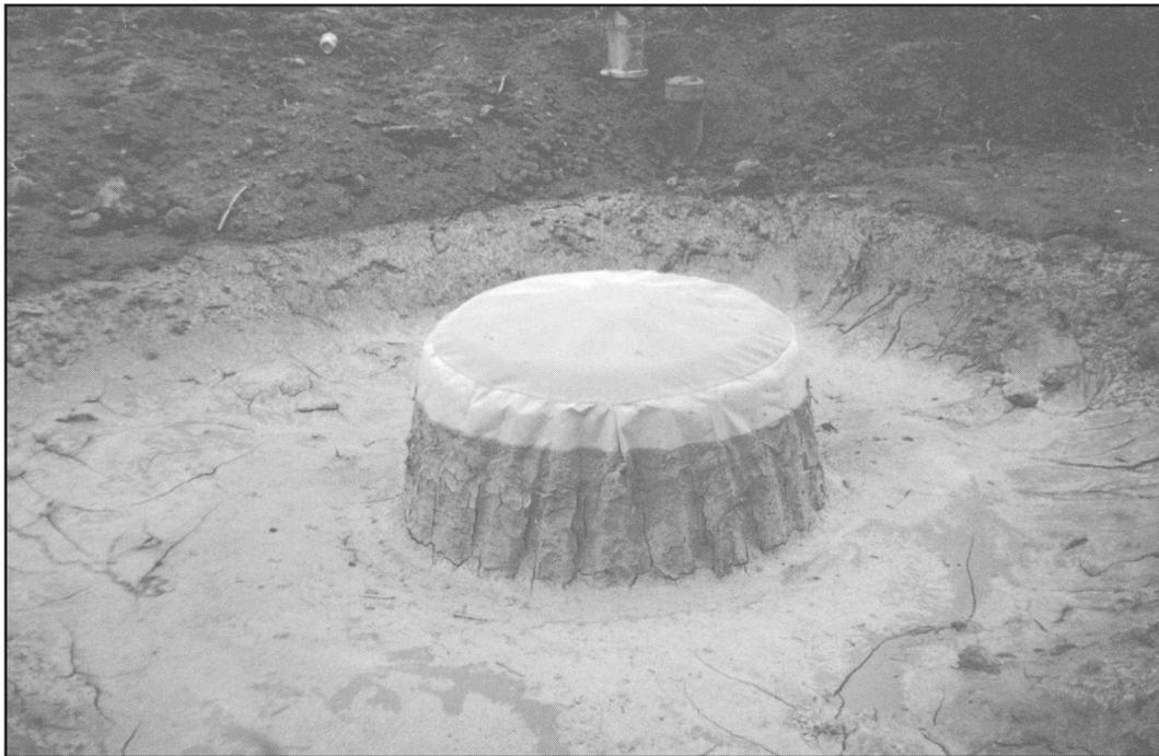
**Figure 6-28.7 Equivalent Inlet Sediment Trap**
